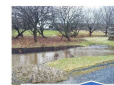
Example of water being contained in a bio-retention area after rain event.
