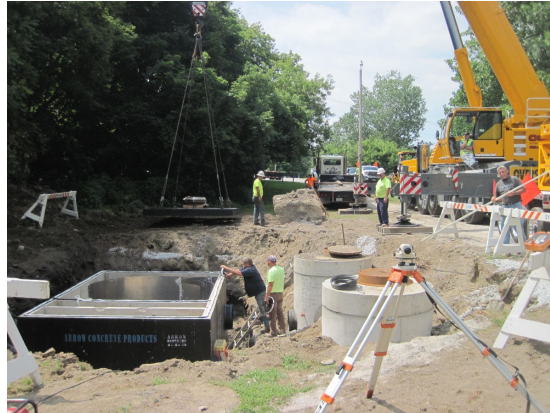
Contech Vortechs Unit being installed in Swanton, VT Summer 2016
