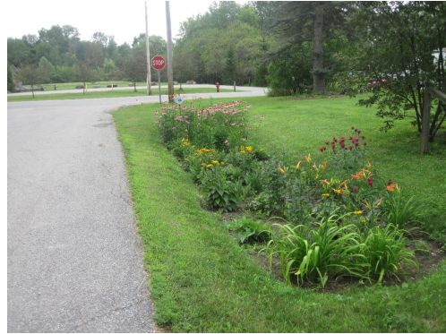
Swale with Raingarden, Woodbine Road, Shelburne, 2017
