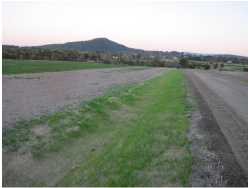
Reconstructed grass swale, East Thompson Point Road, Charlotte, Vermont, Summer 2016
