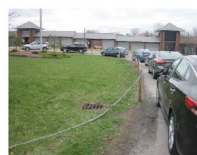
Figure 4: The entrance island at the front of the school has been identified as a possible location for a bio-retention area.
