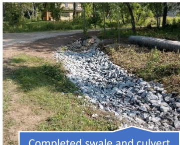
Completed swale and culvert replacement east of Big Oak Lane
