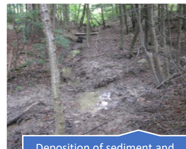
Deposition of sediment and nutrients are occurring at the downstream end of the swale
