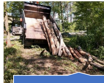
Logs about to be installed in gully as check dams
