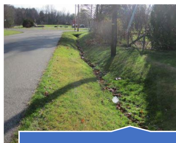
Erosion along deep narrow swale
