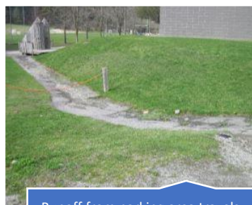
Runoff from parking area travels down the path, carrying sediment and causing erosion
