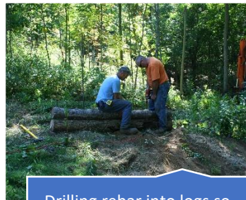
Drilling rebar into logs so they stay in place
