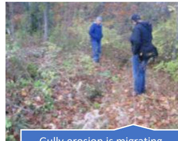
Gully erosion is migrating further to the northeast along the swale
