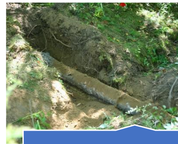
Log jam installation
