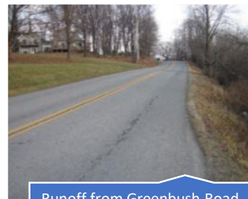
Runoff from Greenbush Road and homes travels through this site to Thorp Brook
