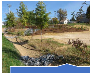
Adjacent completed Silver Street rain garden
