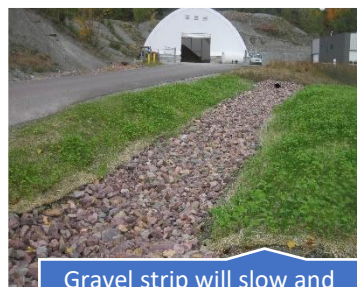
Gravel strip will slow and spread water out onto the vegetated floodplain
