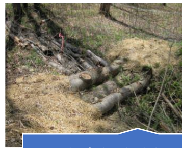
Example of a log check dam and brush log application
