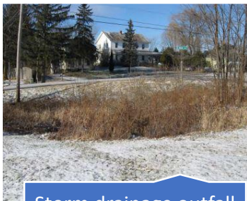
Storm drainage outfall looking east
