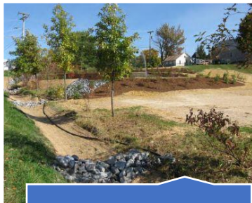
Completed swale and lower treatment looking north
