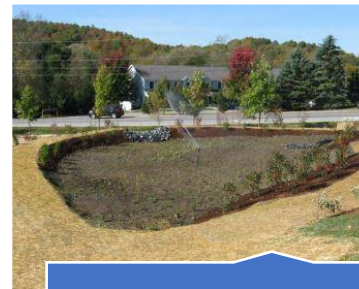
Completed lower bio-retention cell looking west
