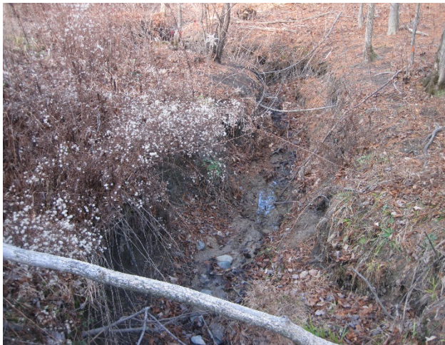
Figure 6: Gully erosion occurring in the channel leaving the neighborhood.
