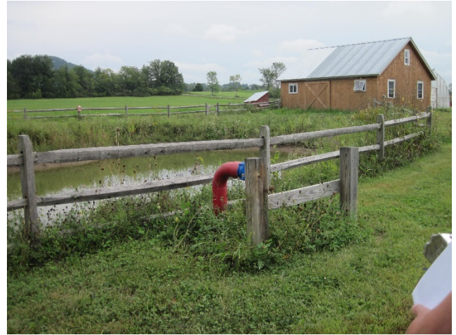
Figure 3: A fire pond is located on the site, but does not have significant stormwater storage capacity.
