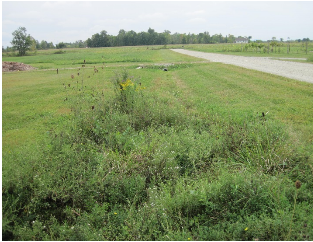
Figure 1: This swale is collecting runoff from the gravel road and field.
