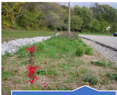
Filter strip off Shelburne Community School parking lot slows down and filters water before it reaches the swale and McCabe's Brook
