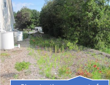
Bio-retention area east of building with rain barrels (where former entrance driveway was)
