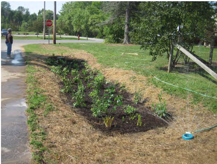
Project construction and planting complete.
