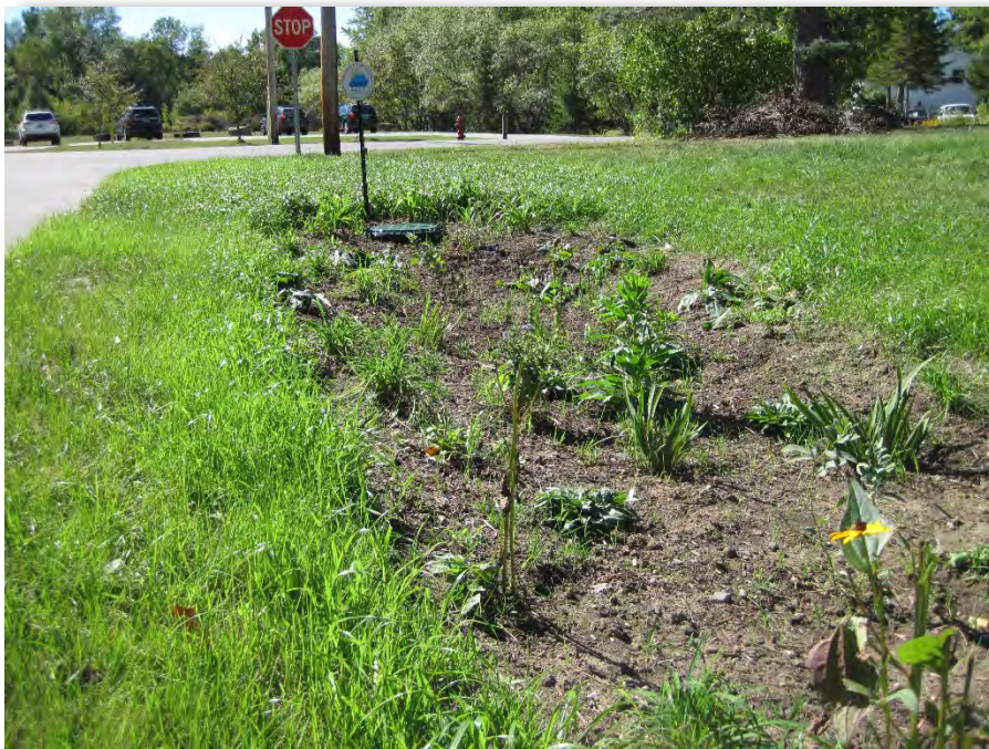
Post-Construction, September 21, 2016: Raingarden created and planted.
