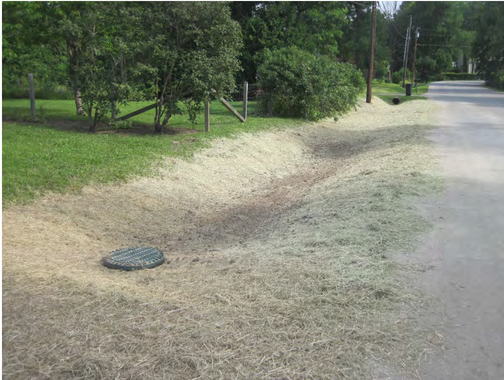
Site view at raingarden area, ready for planting.
