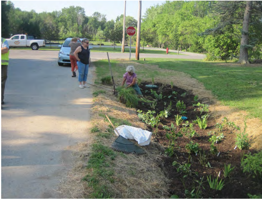
Raingarden area, planting almost complete.
