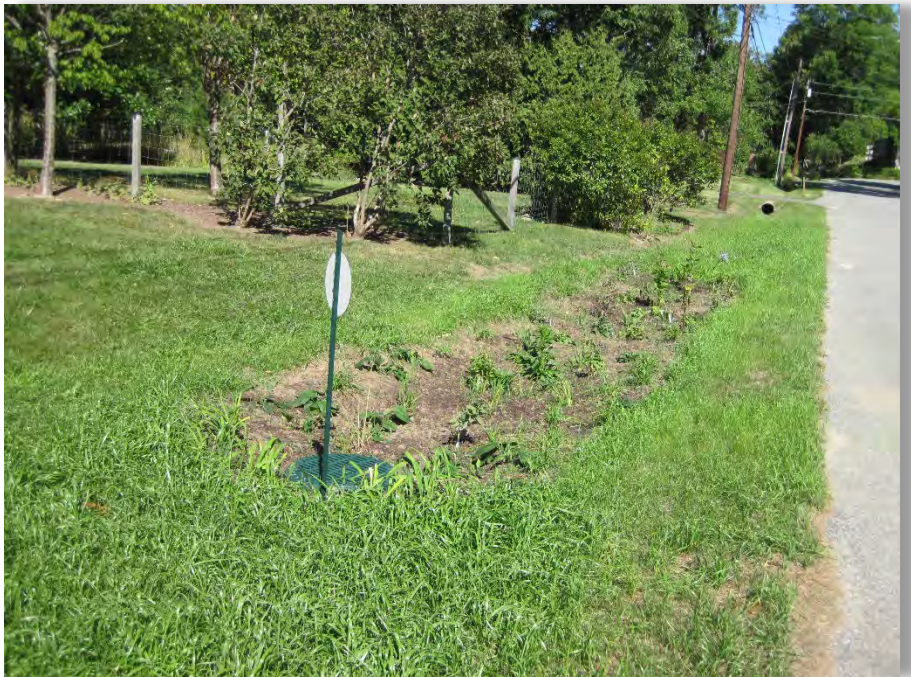
Post-Construction, September 21, 2016: Raingarden created.
