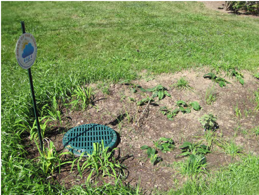
A close view of the plants, Ahead of the Storm signage, and stormwater inlet at the downstream end of the final raingarden, viewed looking west from Brook Lane.
