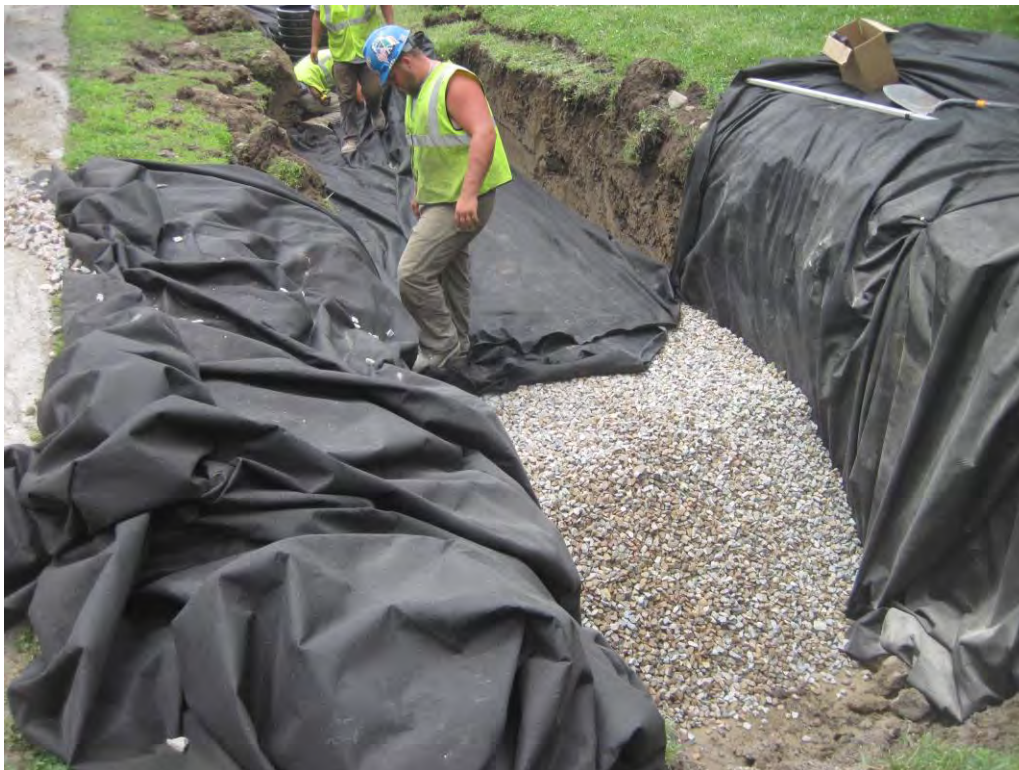
Gravel and geotextile fabric under raingarden section in progress.
