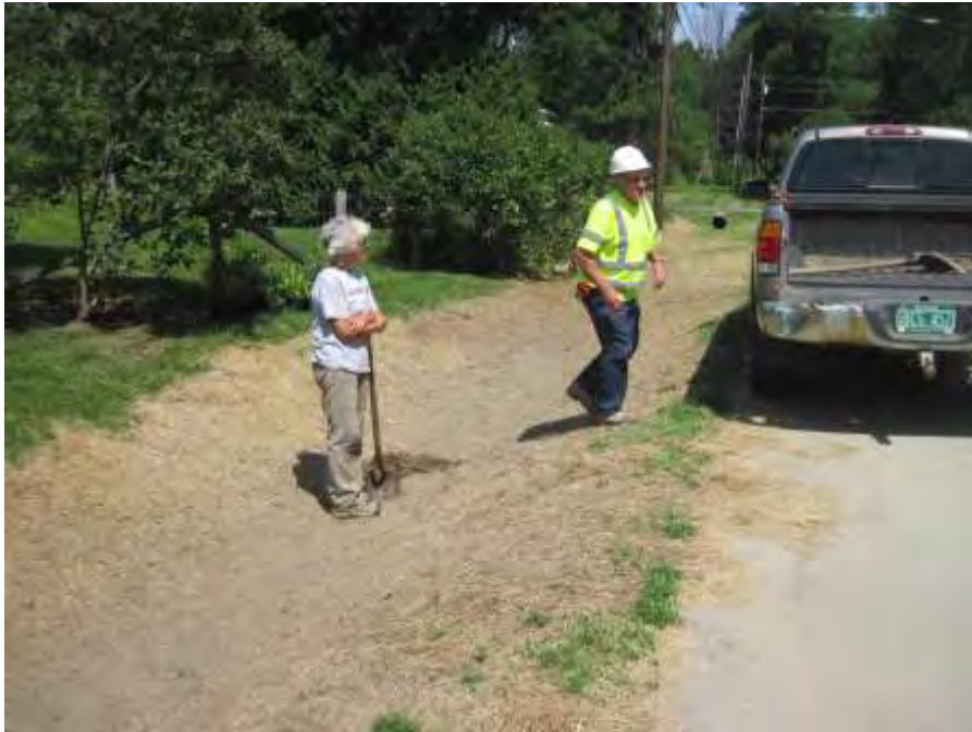
Raingarden area is ready for planting.
