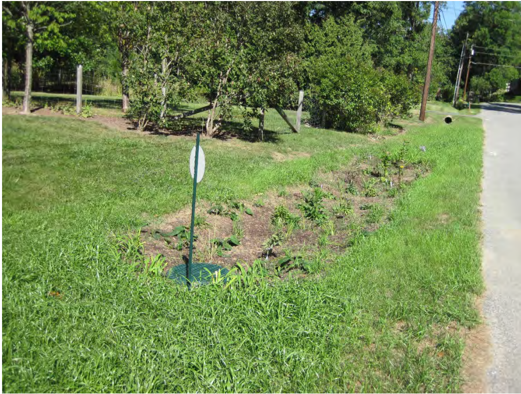
The final raingarden, viewed looking north along Brook Lane.
