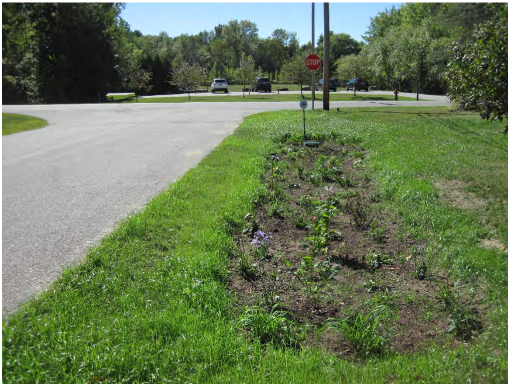
The final raingarden, viewed looking south along Brook Lane. The planting medium, infiltration trench, and perforated pipe are located below ground.
