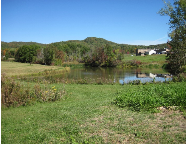
Figure 1: Existing fire pond provides treatment for water quality, channel protection, and Q10 and Q100 attenuation (Recommendation 5).
