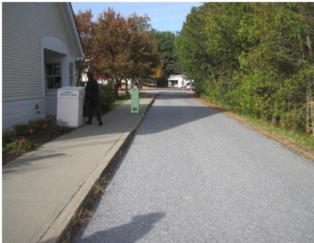
Figure 2: Library entrance driveway. Existing site runoff sheet flows across driveway to swale on other side in bushes.
