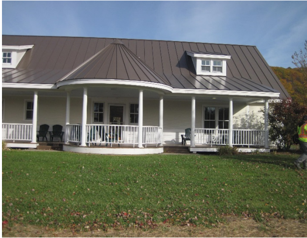
Figure 5: West side of the library. Roof runoff currently falls off roof and travels overland into the Green.
