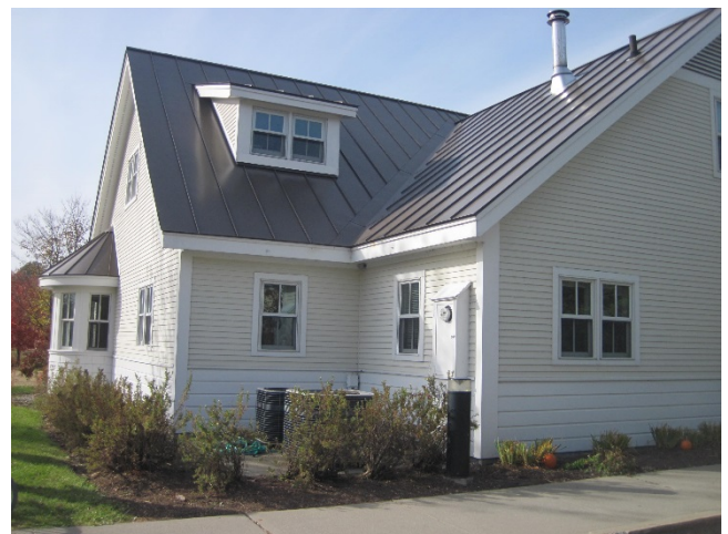
Figure 4: Potential location of new gutter, downspout, and rainbarrel to be used for garden watering.
