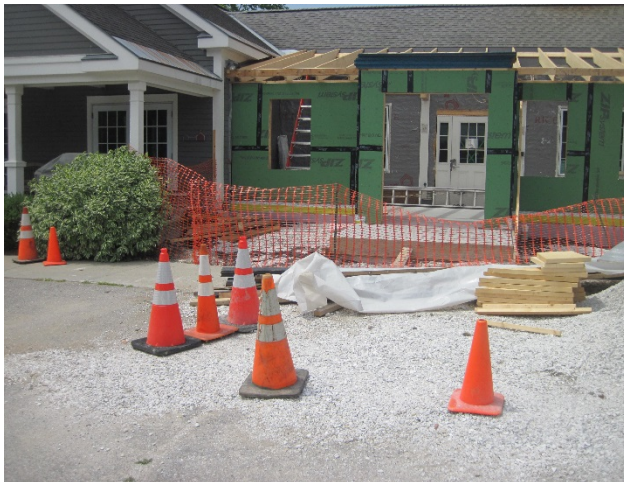
Figure 2: Senior Center existing entryway, in process of being expanded.
