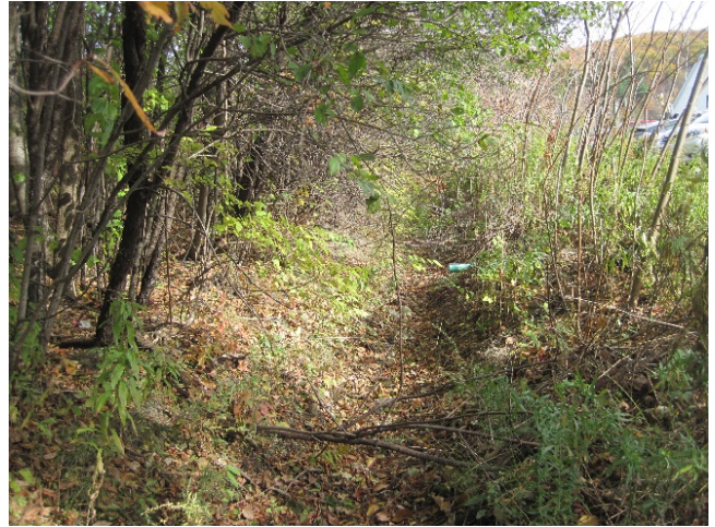
Figure 7: Swale at the north side of property, with some erosion visible.
