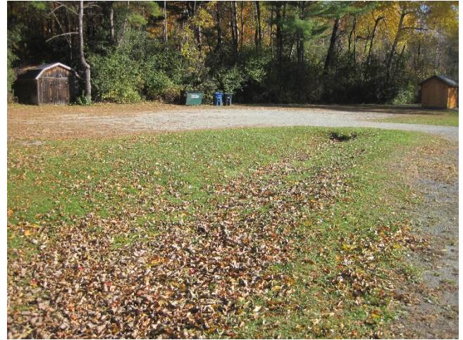
Figure 7: A swale carries water from the parking area and cemetery to the east and into the wetland.
