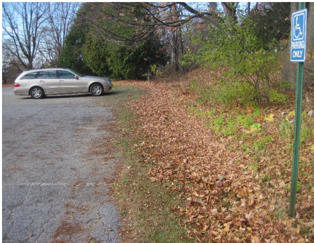
Figure 6: A swale carries water from the parking area and cemetery to the east and into the wetland.
