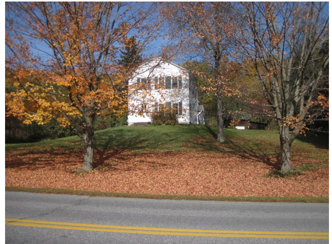
Figure 11: A portion of the parsonage property drains to the roadside swale and eventually flows through a culvert under Church Hill Road.
