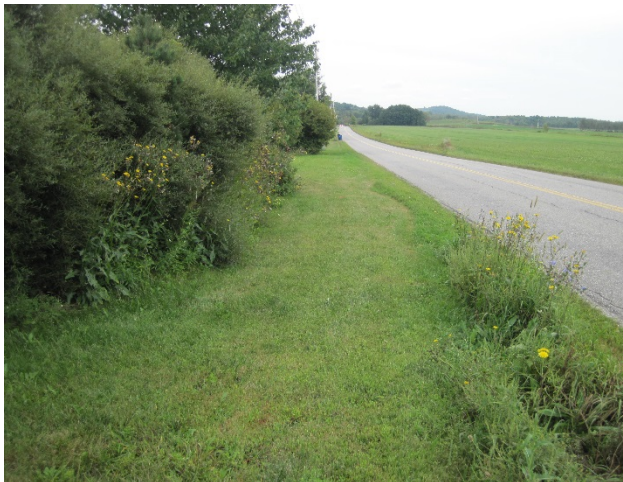
Figure 2: In front of the Du Brul residence, some water continues down swale along the road.
