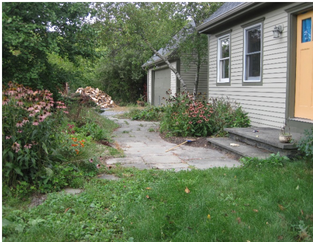
Figure 6: The ground in front of the entryway is low.
