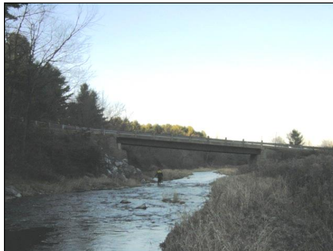
Figure 6.4. M10 Bridge at Carpenter Rd.
