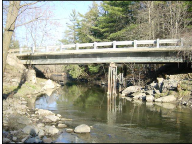
Figure 6.5. M11 Bridge at Dorset Street
