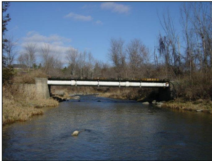
Figure 6.2. Farm access bridge in M06.
