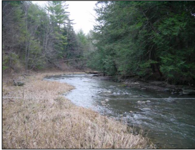
Figure 6.12. View of reach M9A upstream of Spear Street with small floodplain terrace developing.
