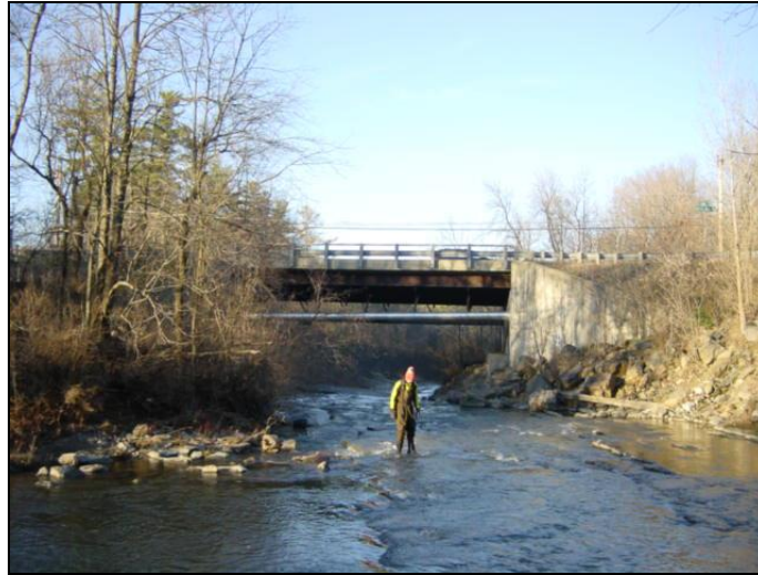
Figure 6.1. Shelburne Falls Road Bridge in M05.
