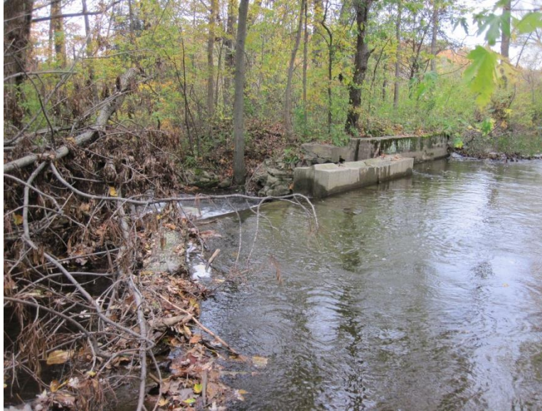
Photo 1: Diversion structure along Patrick Canal at T4.02, looking upstream along Canal.
