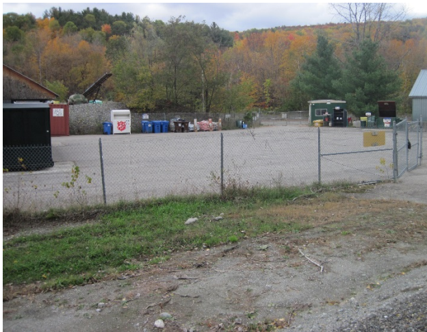
Figure 6: CSWD operates a Drop-Off Center including a paved area and buildings.
