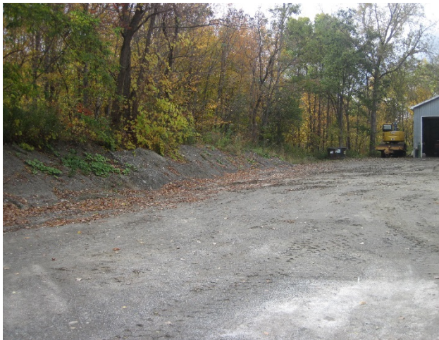
Figure 2: A berm exists between the Garage staging area and Beecher Hill Brook.
