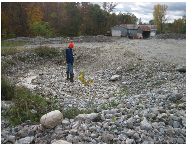
Figure 7: Depressions have been created around the site to capture runoff.
