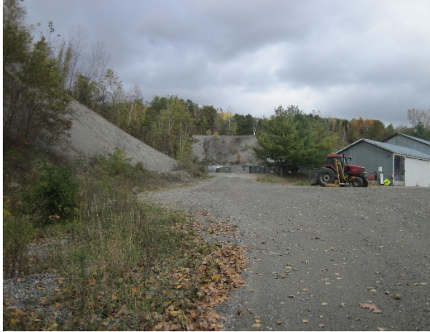
Figure 5: Depressions have been created around the site, including adjacent to the access road to catch water.
