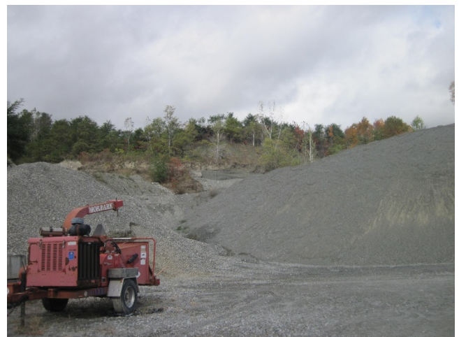
Figure 4: Active excavation in the gravel pit area also includes large piles of stored gravel.
