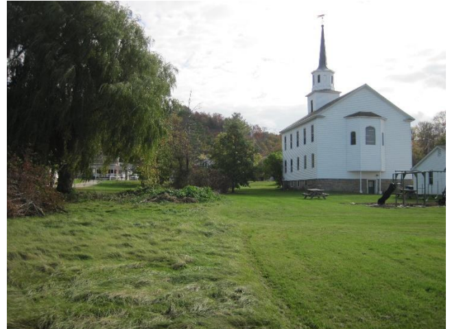
Figure 19: North edge of mowed lawn area looking east. Piles near ditched swale turn visible on image left (October 6, 2020).
