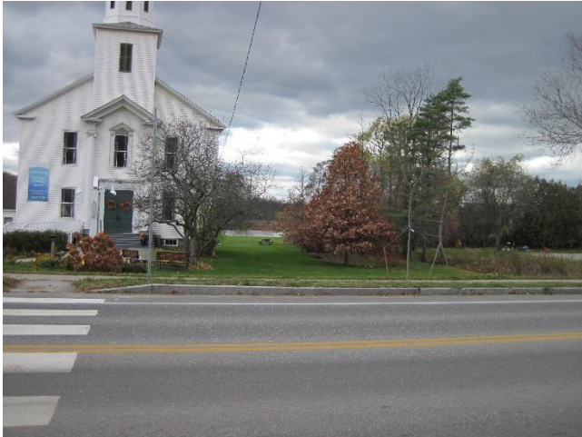
Figure 1: United Church of Hinesburg looking west with culvert outlets and ditched swale shown on the right side of this photo and Route 116 in the foreground (November 1, 2019).
