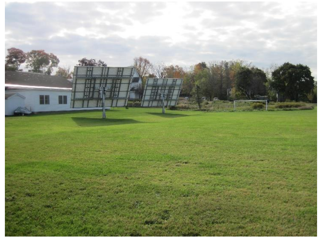
Figure 20: Wetland at image right with wetland finger extending into swale along solar panels (October 6, 2020).
