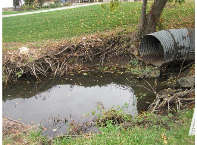
Figure 3: Outlet of 36 inch corrugated metal pipe under Route 116 (October 6, 2020).
