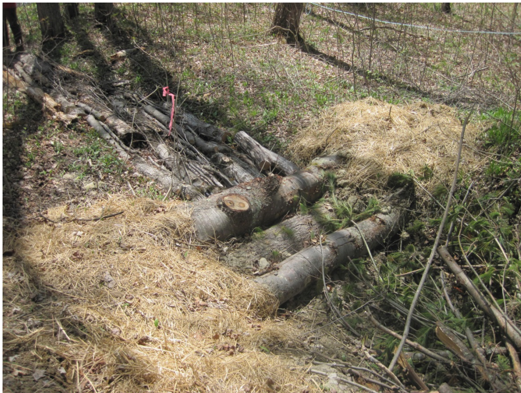
Photo 2. Example of log check dam and brush and small log application at gully erosion site adjacent to Pond Brook in Monkton, Vermont. This photo was taken at time of installation, prior to accumulation of sediment between the logs and brush.
