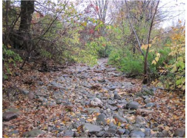
Figure 3: Hollow Brook has been straightened and is dry portions of the year downstream from the culverts where deposited sediment has filled in the channel bed (October 2, 2020). The channel was observed flowing October 28, 2019 and December 6, 2020 and observed dry August 3, 2020, October 2 and 9, 2020.
