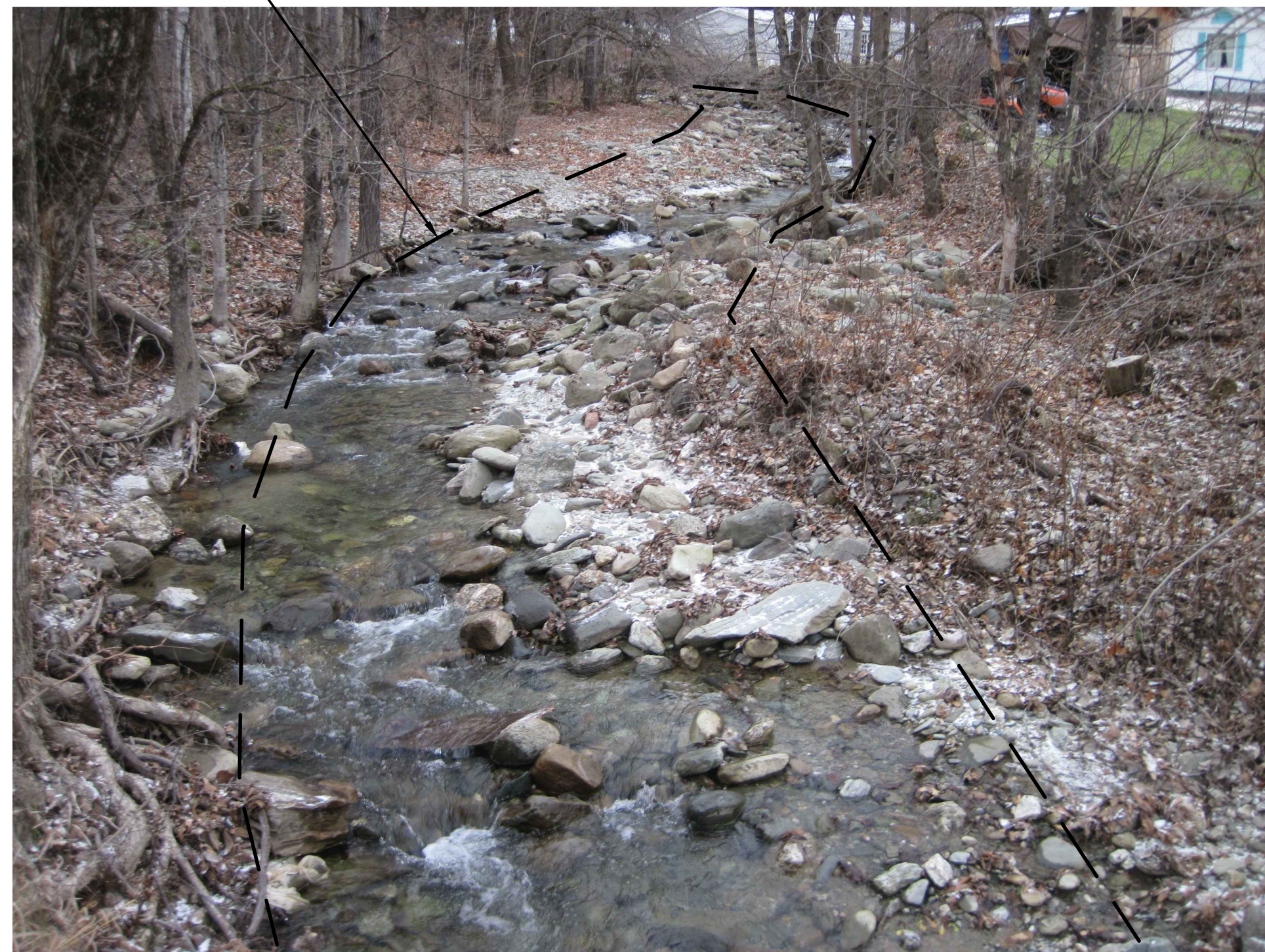
SEDIMENT REMOVAL IMMEDIATELY UPSTREAM OF CULVERTS
