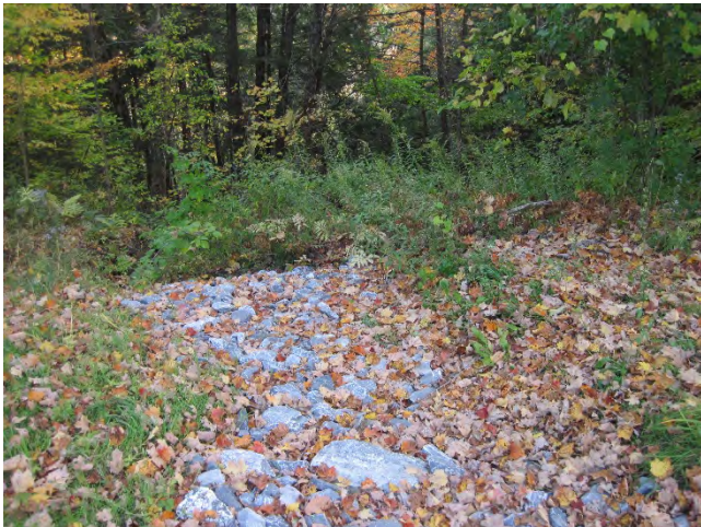
Figure 18: Stormwater from Lincoln Hill Road flows over erosion stone and then enters to top of the steep gully channel (October 9, 2020).
