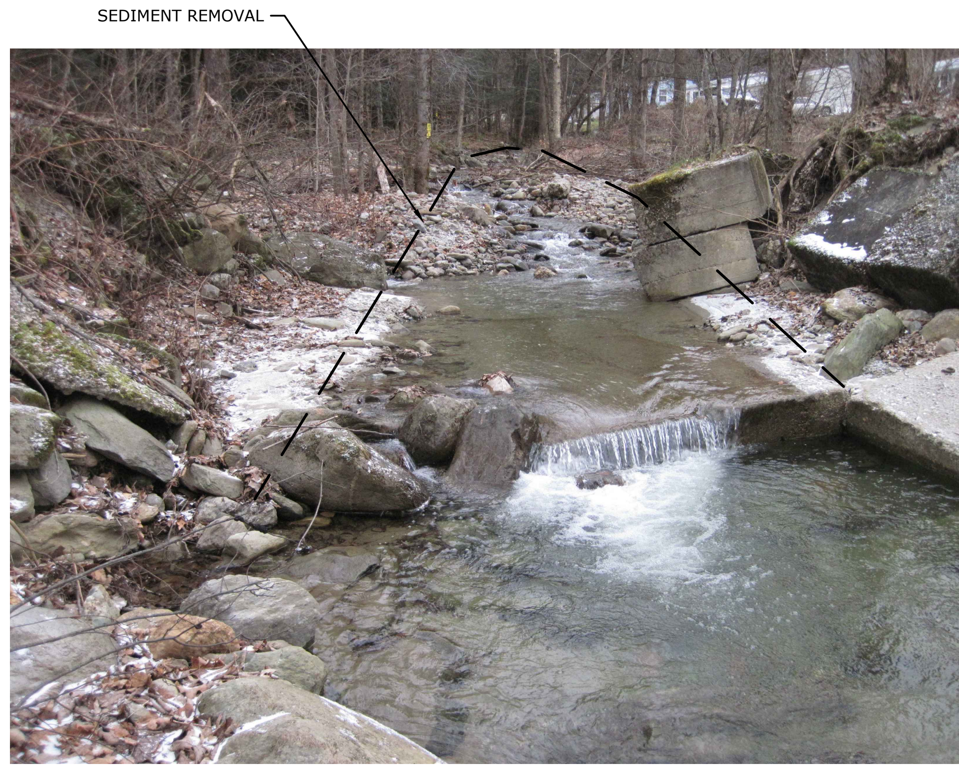
SEDIMENT REMOVAL OLD BRIDGE
