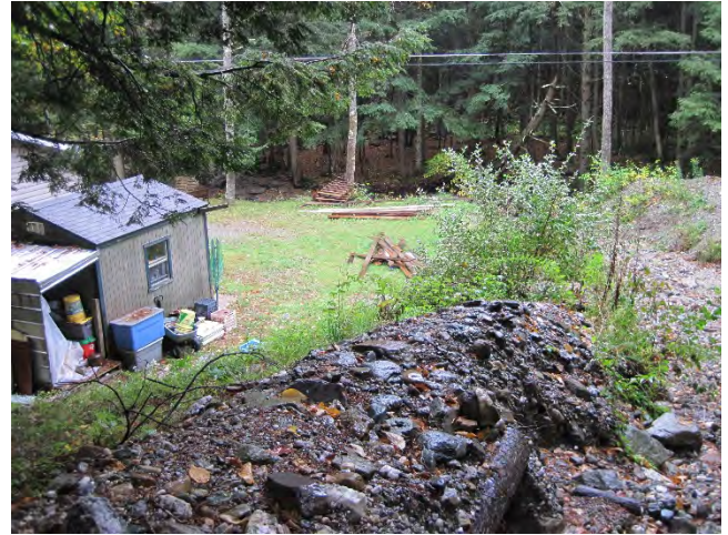
Figure 20: Runoff from uphill along Lincoln Hill Road flows down this steep tributary, contributing large amounts of sediment which have been cleaned out often and now bermed up to protect nearby home (October 2, 2020).
