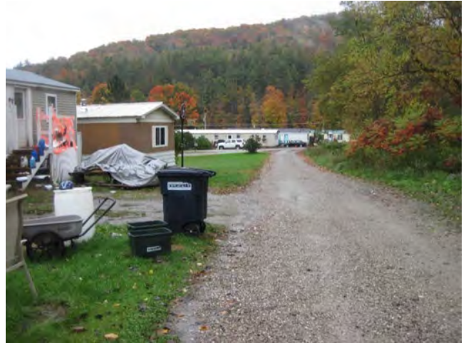
Figure 23: Many homes along Elm Lane and Lazy Brook Drive are vulnerable to damages from inundation or sediment deposition. Several have already experienced damages (October 2, 2020).
