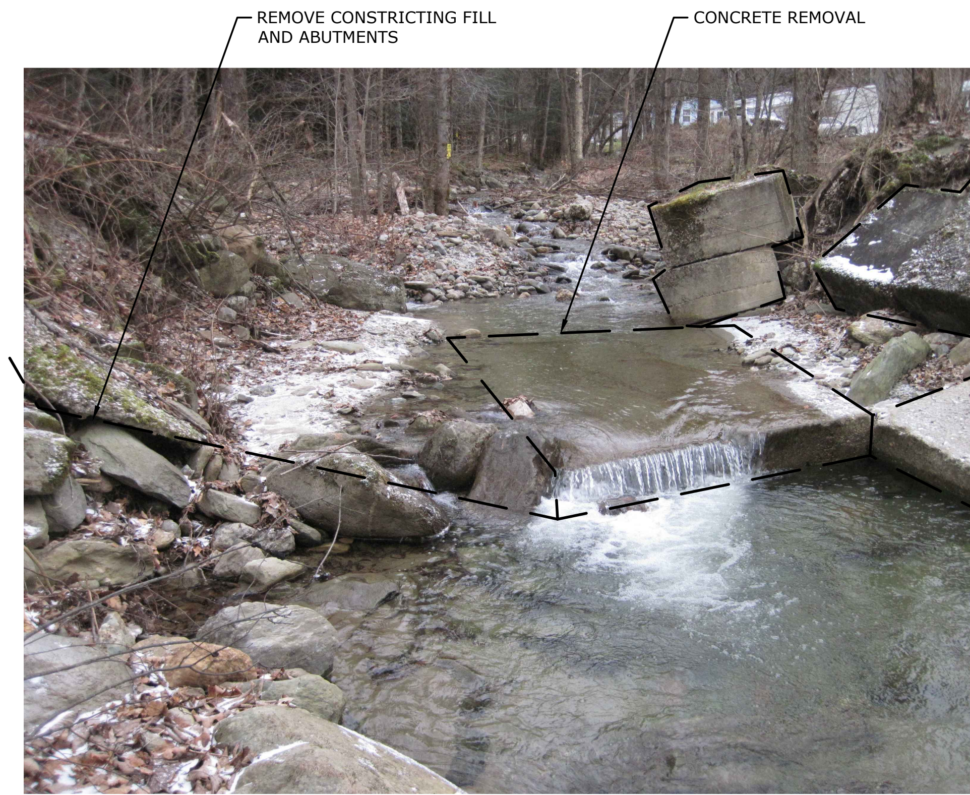
CONCRETE, FILL, AND ABUTMENT REMOVAL OLD BRIDGE
