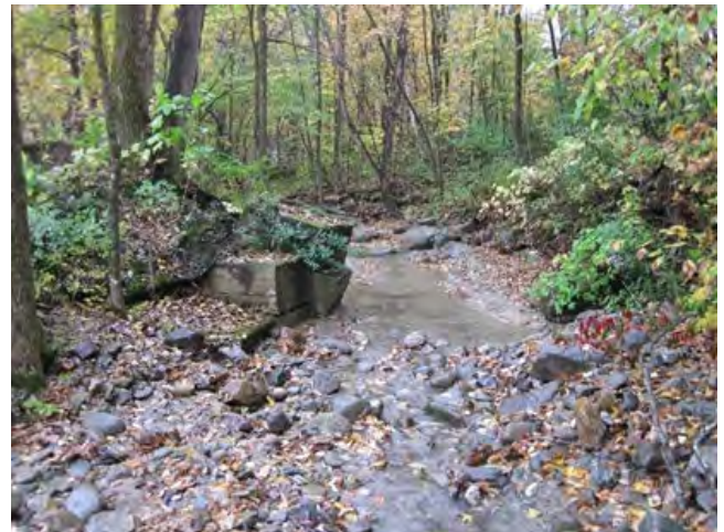
Figure 16: View of old bridge abutments looking downstream (October 2, 2020).
