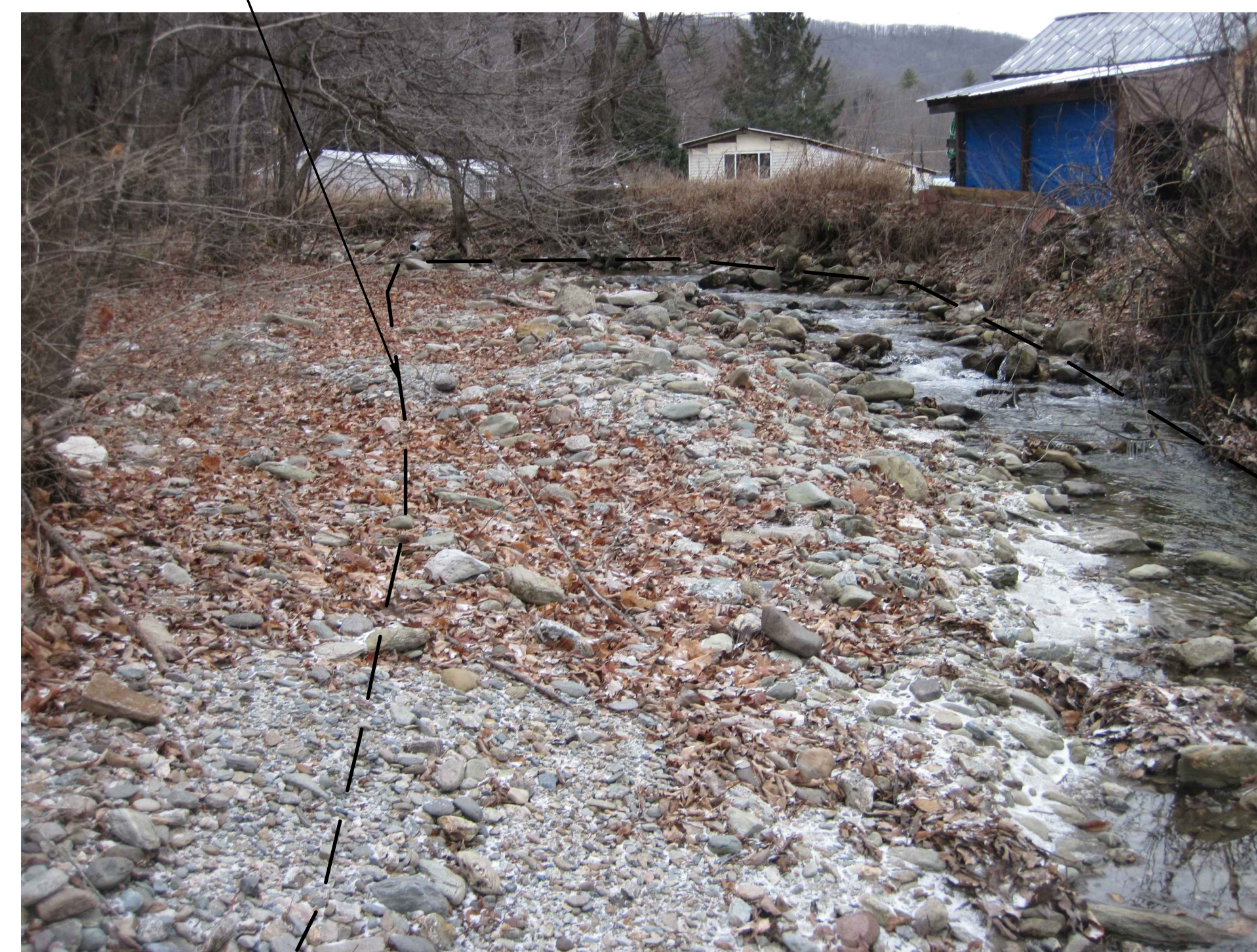
SEDIMENT REMOVAL AT UPSTREAM END OF CULVERT AREA
