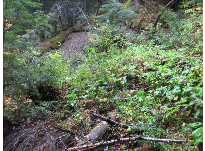
Figure 26: Upstream mass failures naturally healing with vegetation (October 2, 2020).
