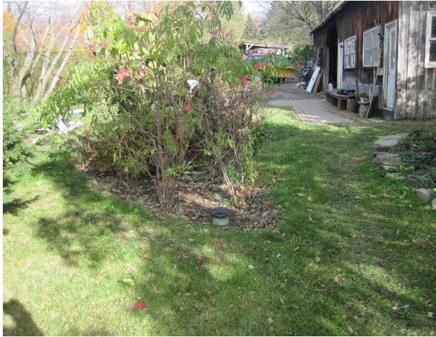
Figure 5: A small raingarden was installed to catch sediment leaving the loading area.
