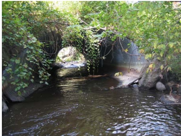
View upstream to culvert outlet
