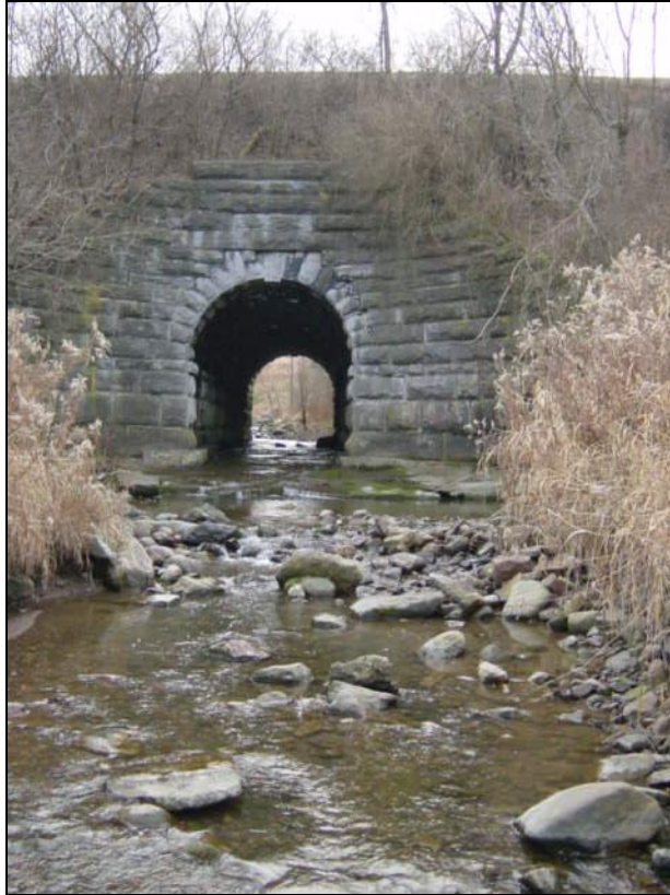
Railroad crossing on T1.05A from downstream looking upstream.
