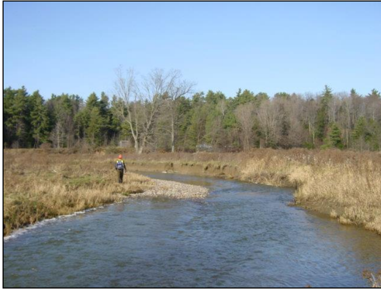
Right bank erosion and diagonal bar.
