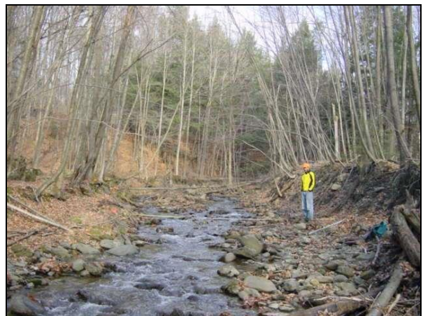
Significant channel enlargement following straightening and berming.
