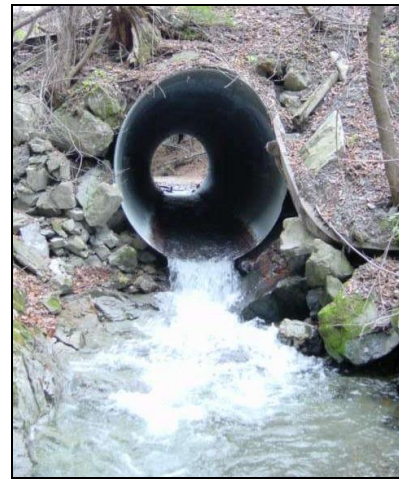
Beecher Hill Brook (T5.01B) culvert. Note aggradation forming bars and splitting flow upstream. Some erosion was noted downstream, although the downstream end falls onto ledge and boulders.
