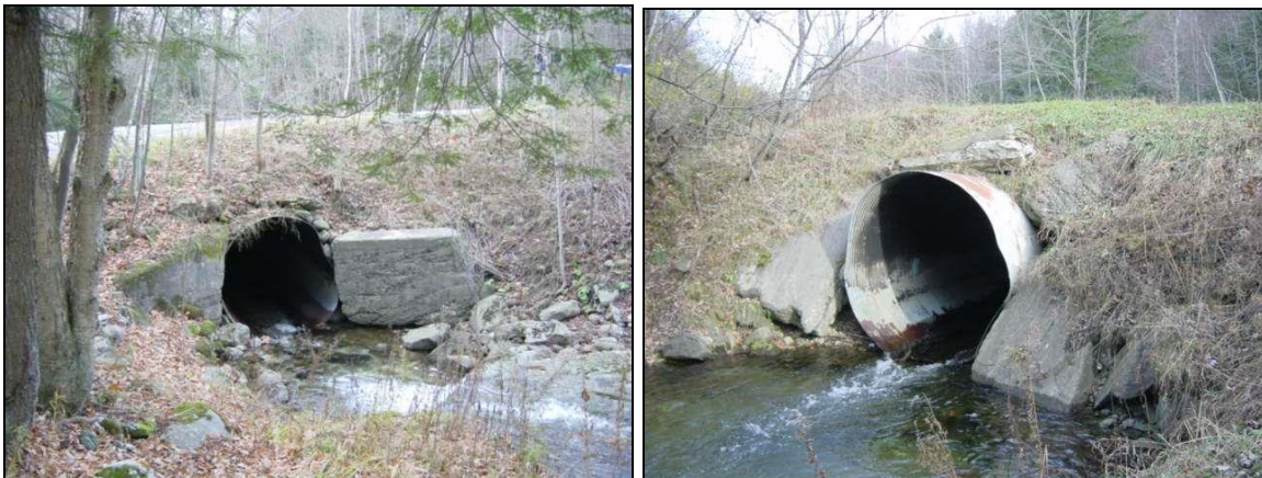
Culvert at North Rd views: upstream end and downstream end.
