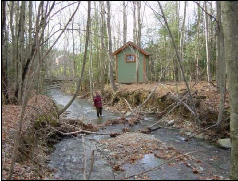
Channel enlargement further downstream leaving investments in danger.
