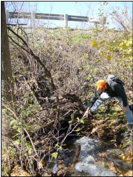
Culvert on segment M18B. The upstream end of the culvert was blocked by sediment and debris and was hardly visible (left). Extreme scour was apparent at the downstream end and beyond (right).
