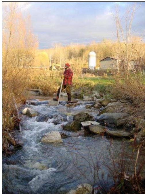
Headcut downstream of Beecher Hill Rd.
