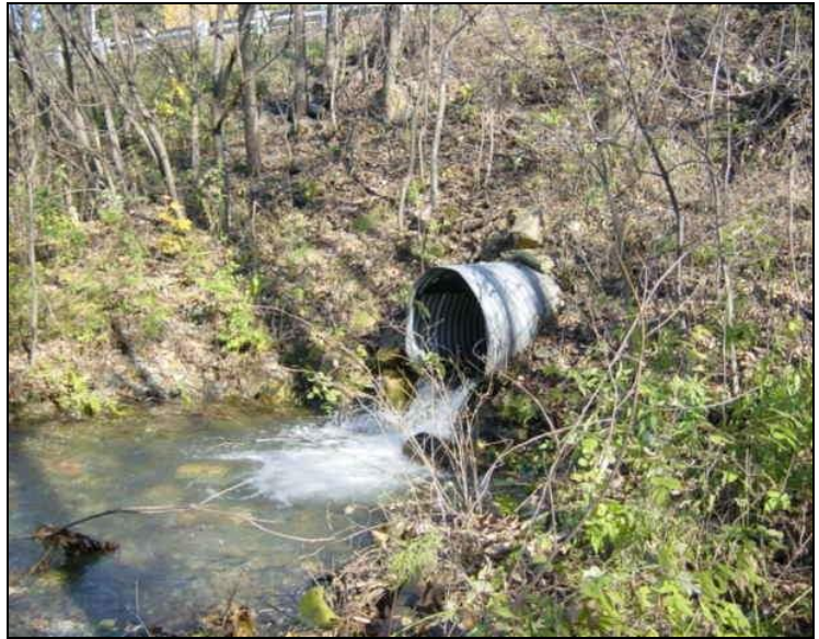
Culvert on segment M18B. The upstream end of the culvert was blocked by sediment and debris and was hardly visible (left). Extreme scour was apparent at the downstream end and beyond (right).
