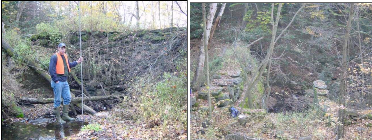
Old mill dam upstream and downstream photos.
