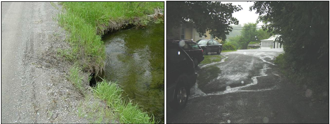
Sand and gravel from roads and driveways washing into the channel.
