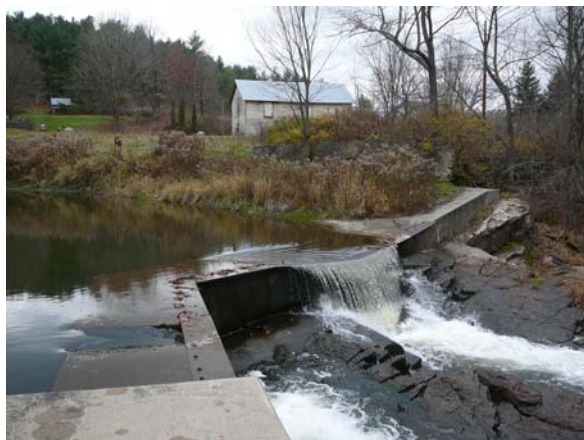
Figure 20. Scott Pond Dam on Lewis Creek segment M09-B.
