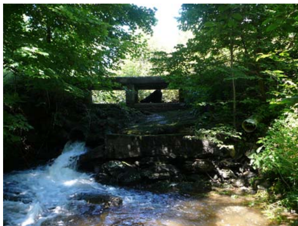
Figure 19. Culvert / dam on Hollow Brook segment T4.05-D.
