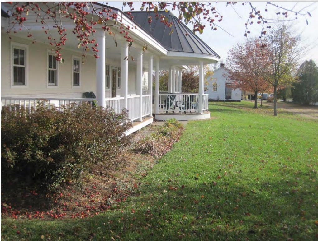
Pre-Construction, October 27, 2015: Porch area facing the Green.
