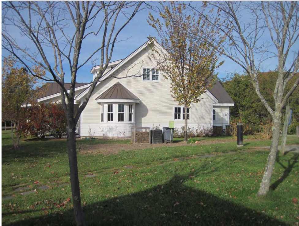
Pre-Construction, October 27, 2015: South end of library building. Existing gardens in foreground could be watered using collected rainwater.
