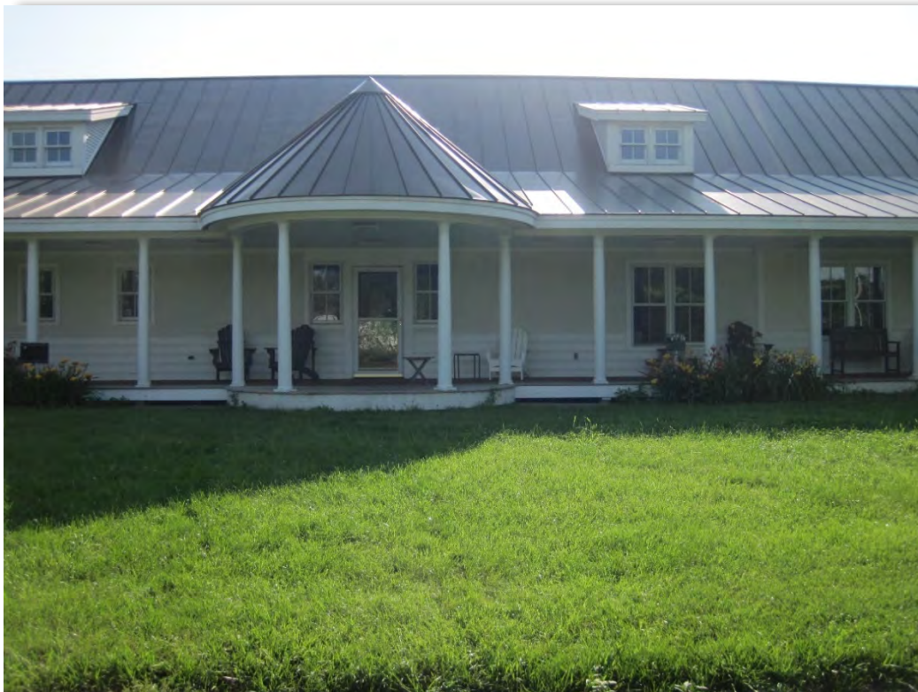
Post-Construction, July 23, 2021: West side of the library. Bio-retention areas planned in front of the porch.
