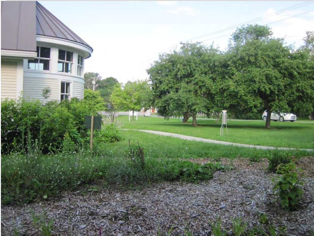
Post-Construction, July 23, 2021: North end of library viewed from the east. New sidewalk has been added providing pedestrian access from Ferry Road. A NOAA rain gage is located at the north end of the building.
