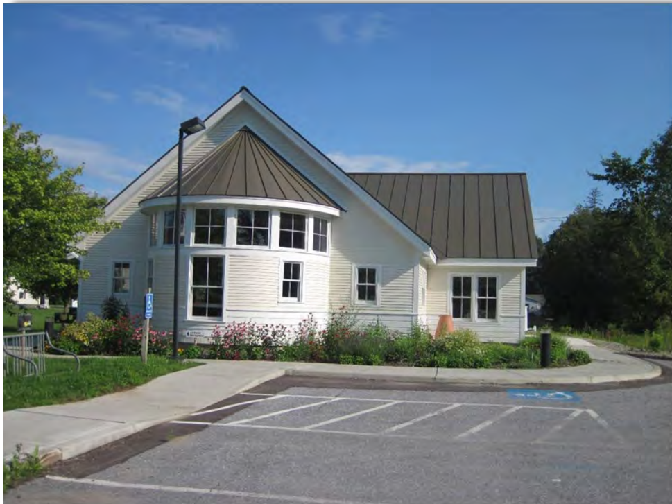
Post-Construction, July 23, 2021: South end of library building. An addition has been added at the south end of the building, rainbarrel installed, and additional gardens planted.
