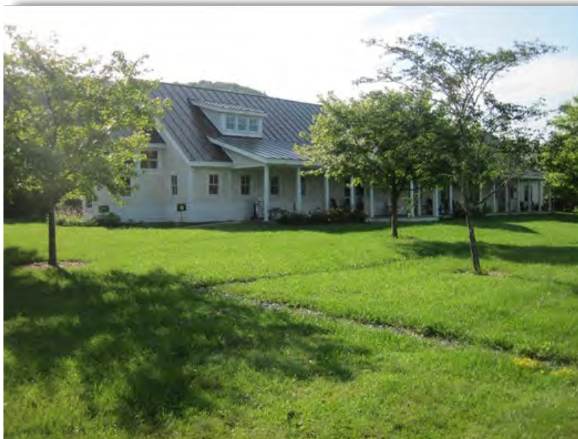
Post-Construction, July 23, 2021: Library building. Railings have been removed. Addition is visible at image right.
