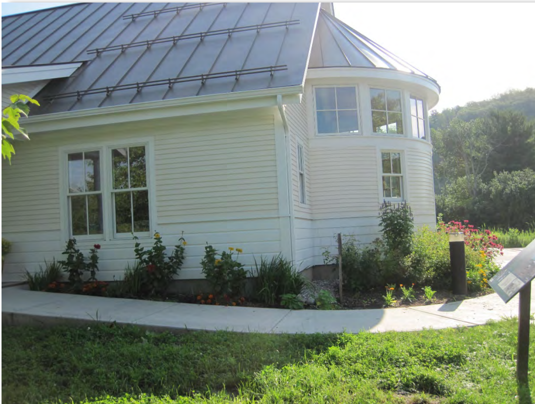
Post-Construction, July 23, 2021: South end of library building addition viewed from the west.
