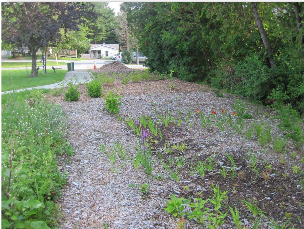
Post-Construction, July 23, 2021: North end of bio-retention area and new sidewalk at former Ferry Road library entrance.
