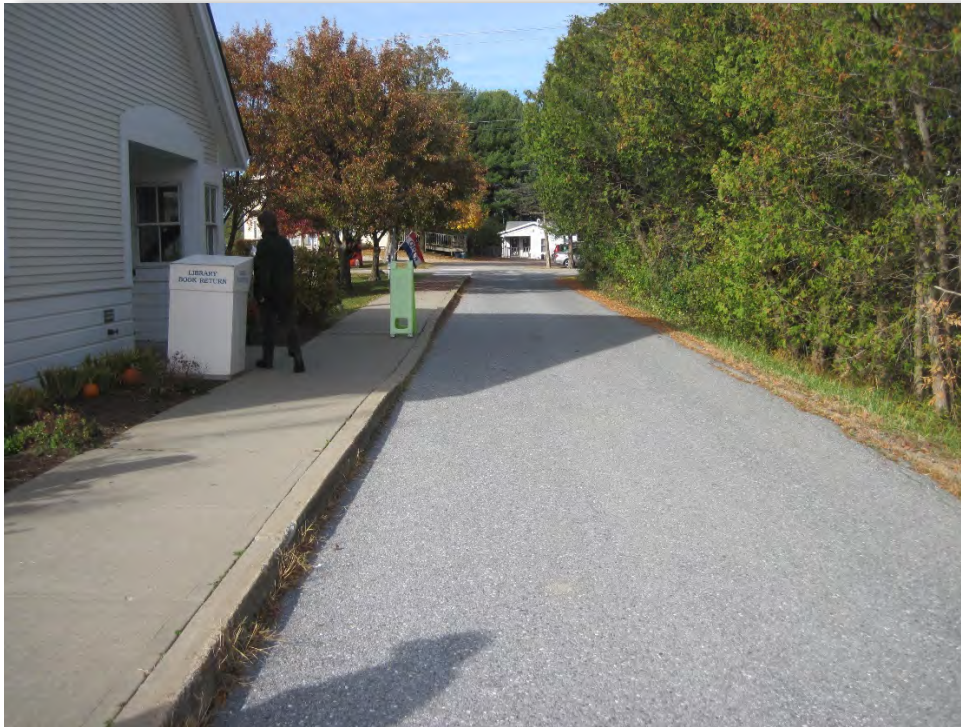
Pre-Construction, October 27, 2015: Library entrance driveway. Existing site runoff sheet flows across driveway to swale on other side in bushes.
