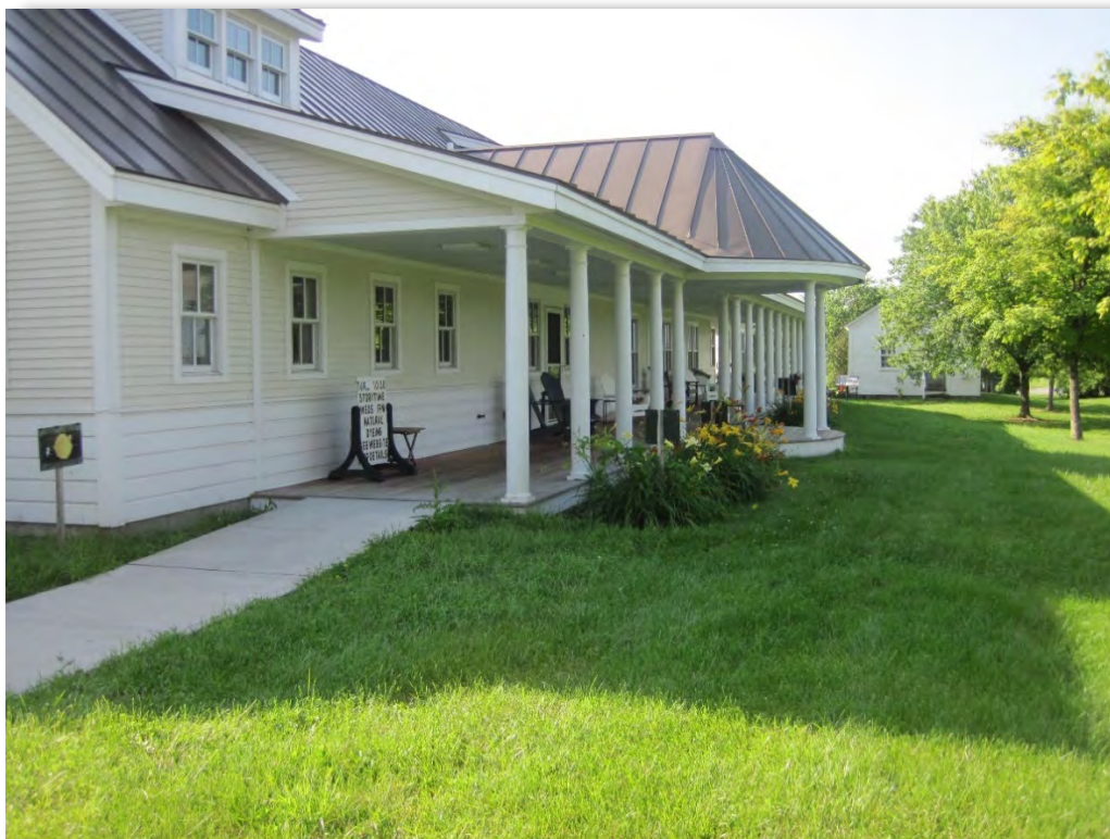
Post-Construction, July 23, 2021: A bio-retention area is planned at this location for a future phase of the project. Runoff from the sidewalk sheet flows into adjacent vegetation as a disconnection practice.
