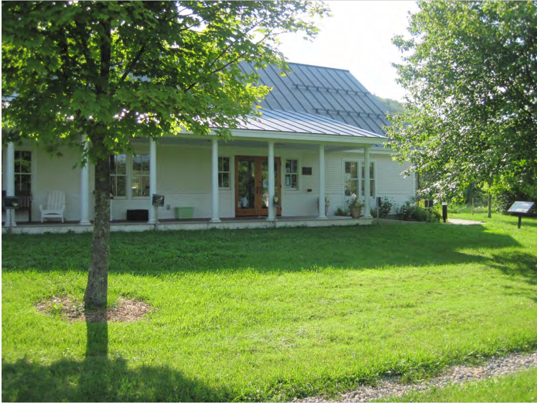
Post-Construction, July 23, 2021: Library building addition viewed from the west.
