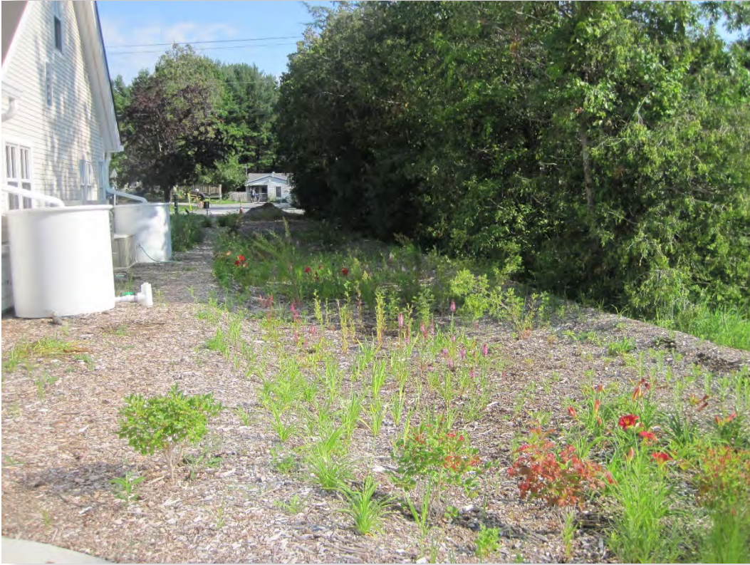
Post-Construction, July 23, 2021: Closer view of bio-retention area and rain barrels.
