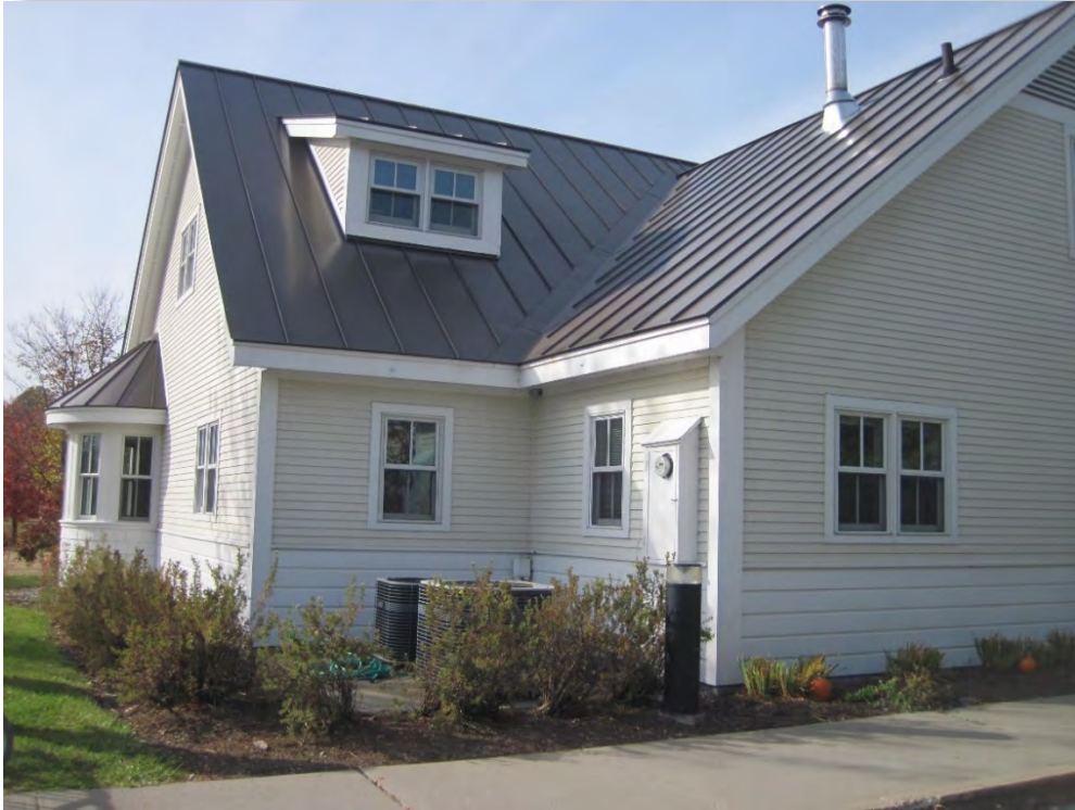
Pre-Construction, October 27, 2015: Pre-expansion end of building.
