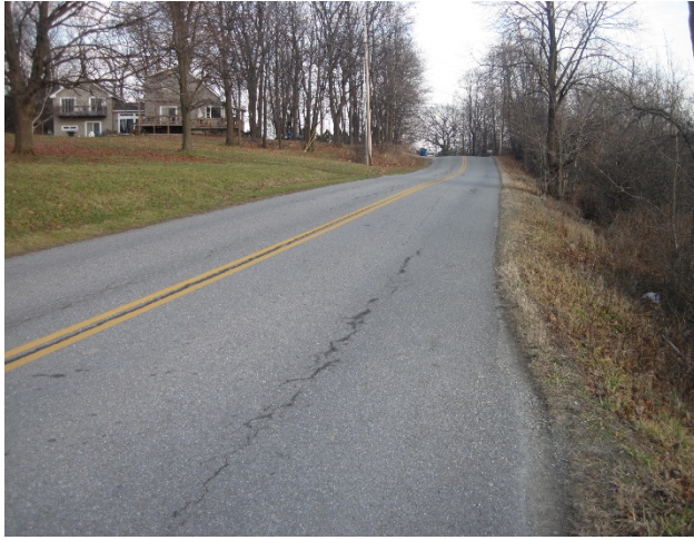
Figure 1: Runoff from Greenbush Road and homes on the far side of the road travels through the adjacent farm fields to Mack's farm field.
