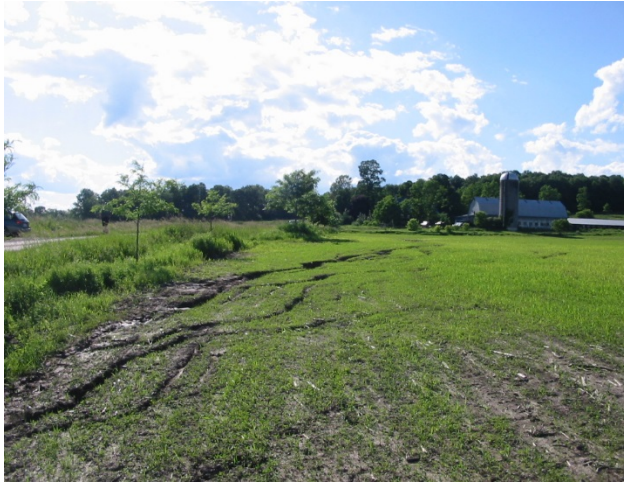
Figure 5: Rill erosion has occurred in the Mack farm field when water in the swale traveling from the north leaves the swale and cuts across the field to the road swale.
