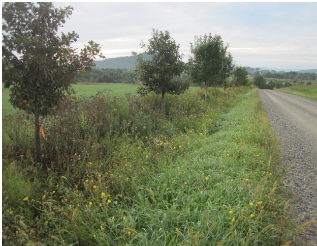
Figure 6: A vegetated swale travels along East Thompson Point Road. The trees in this photo have been moved.
