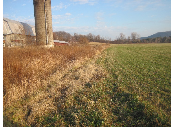
Figure 3: A swale runs from north to south along the west edge of the Mack's farm field, carrying water to the East Thompson Point Road swale.
