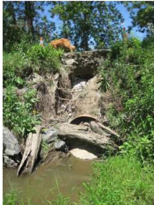
a) b) Photo 5: T1.06A a) typical section and b) failed Lime Kiln Road culvert viewed from upstream end.
