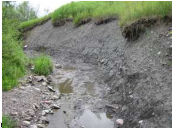
Photo 8: T1.05B a) large mass failure near downstream end a) looking downstream and b) looking upstream.
