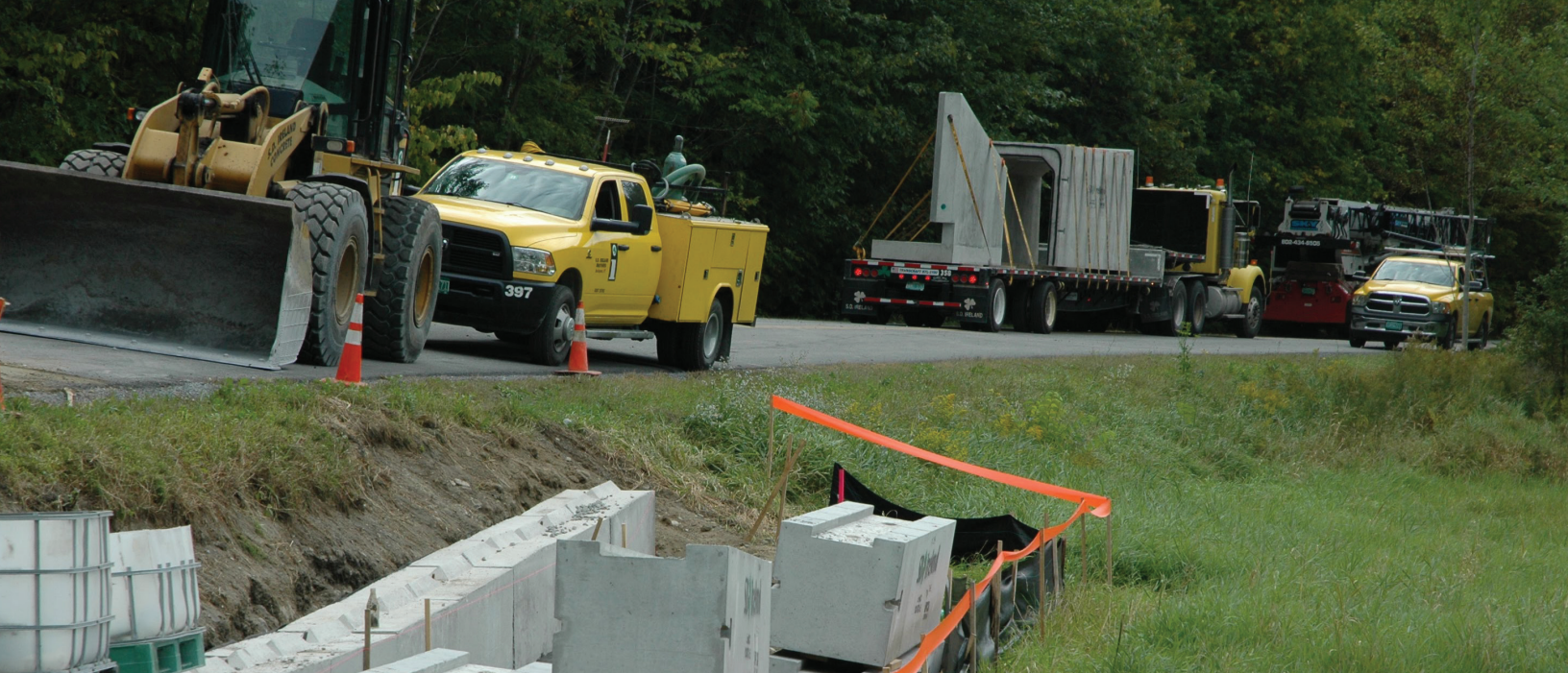
Culvert construction progress. Photo: Chris Slesar
