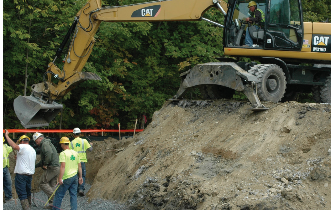
Culvert construction. Photo: Chris Slesar
