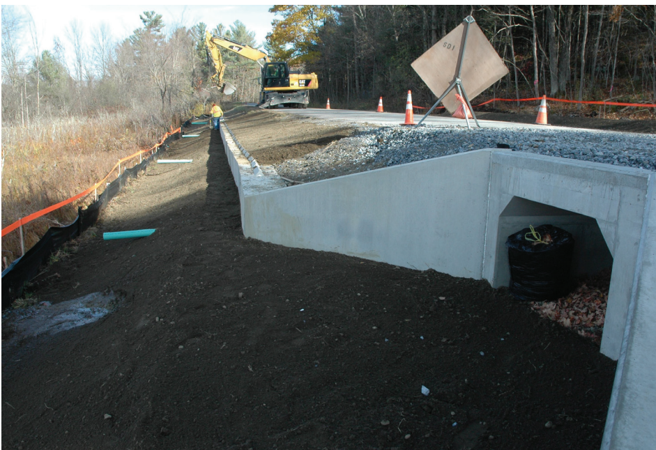
Culvert finalization. Photo: Chris Slesar
