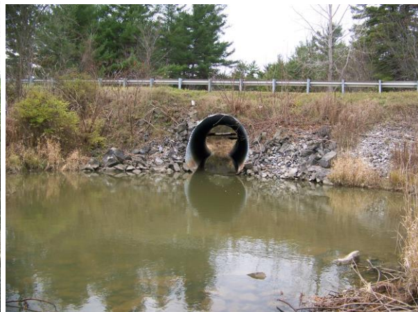
Upstream (L) and downstream (R) views of the southern (upstream) culvert. Note the woody debris upstream and scour downstream.
