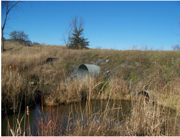
Culverts with overflow pipes (L) and beaver activity (R).
