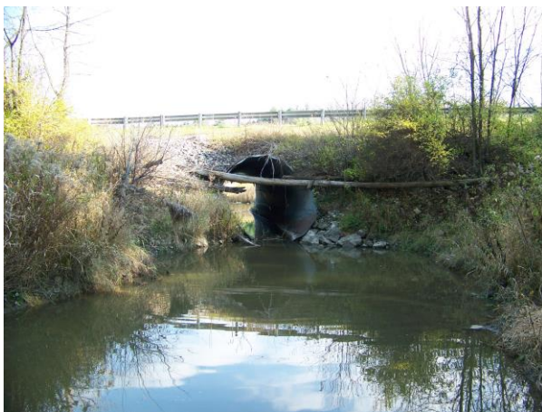
Upstream (L) and downstream (R) views of the southern (upstream) culvert. Note the woody debris upstream and scour downstream.
