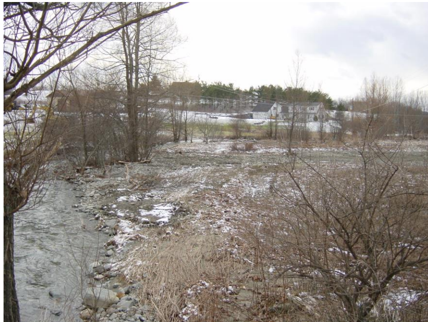
Figure 10. Floodplain fill replaced after January 18, 2006 storm flows, reducing sediment and flow attenuation in this area, which was between 2 degrading areas.
