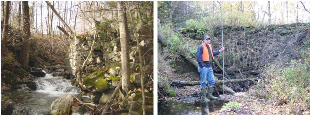
Figure 6. Mill footing on Beecher Hill Brook T5.01C (left) and mill dam on Patrick Brook T4.04 (right).
