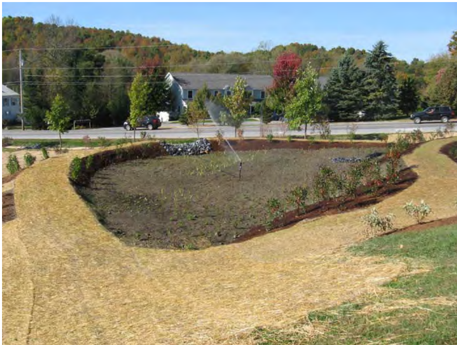
Figure 3: View of completed lower treatment cell.
