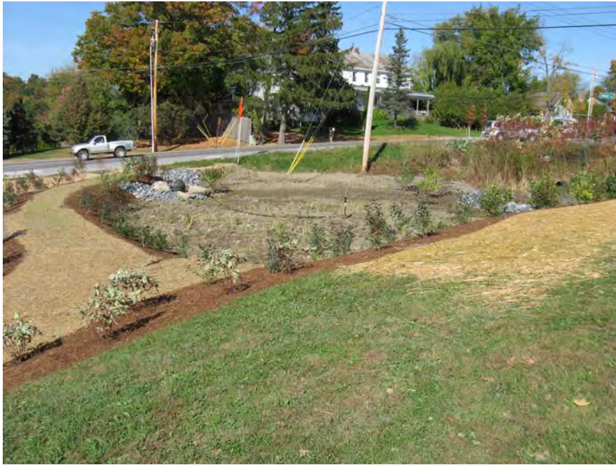
Figure 4: View of completed upper treatment cell.
