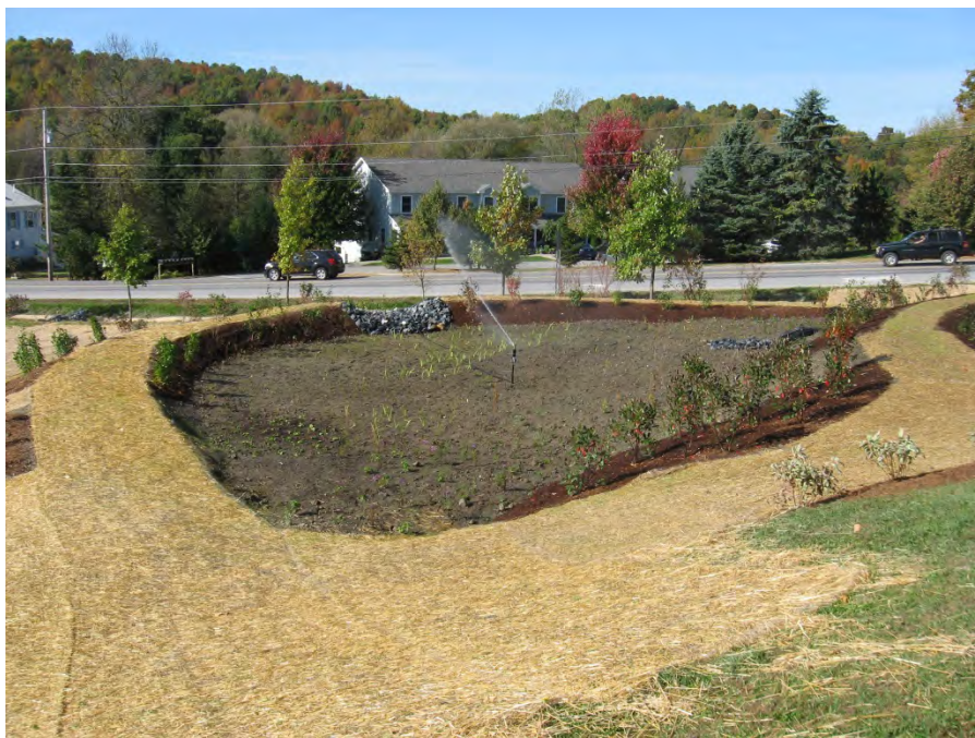
Post-Construction, October 3, 2014: View of completed lower treatment cell looking west.
