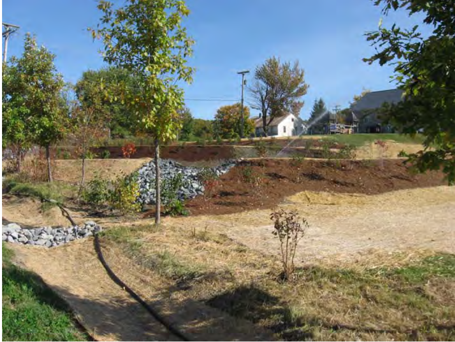
Figure 2: View of completed rain garden treatment cells from Silver Street. Irrigation sprinkler operating in lower cell, and water supply hose visible along the reshaped drainage swale in the foreground. Stone outlet from lower treatment cell and stone check dam visible in the left portion of the photo.
