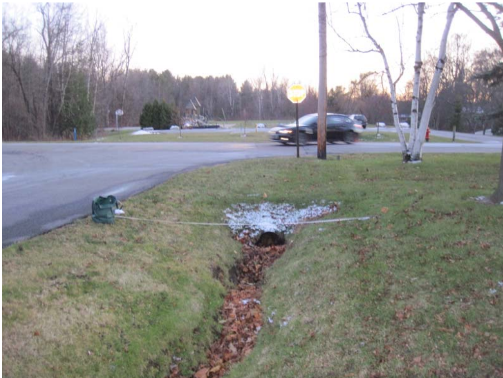
Photo 2: Looking down the Brook Lane swale toward Hullcrest Park.
