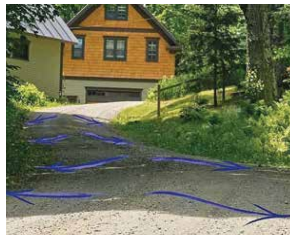
Smooth, crown, and elevate driveways above surrounding land to allow water to run off without eroding the surface.
