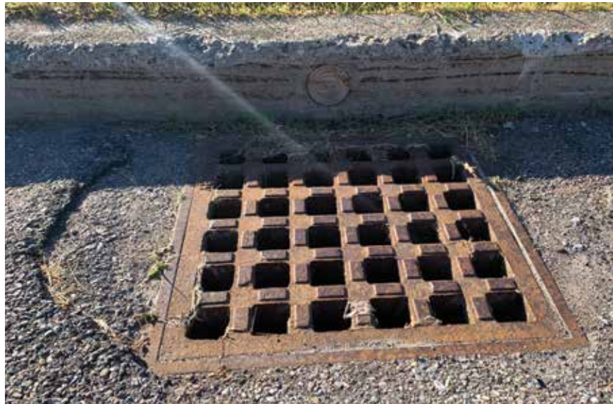
Problem: stormwater and pollutants, like sediment, drain to the Winooski River, with no treatment
