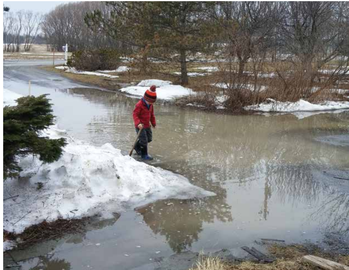
Problem: driveway and garage flood
