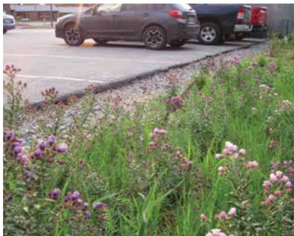
Stone level spreaders allow water that otherwise runs directly off the parking lot into the swale to drop into the stones and spread out.
