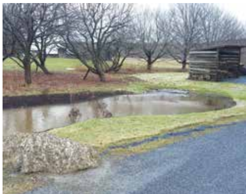
Driveway regraded to direct water to raingarden
