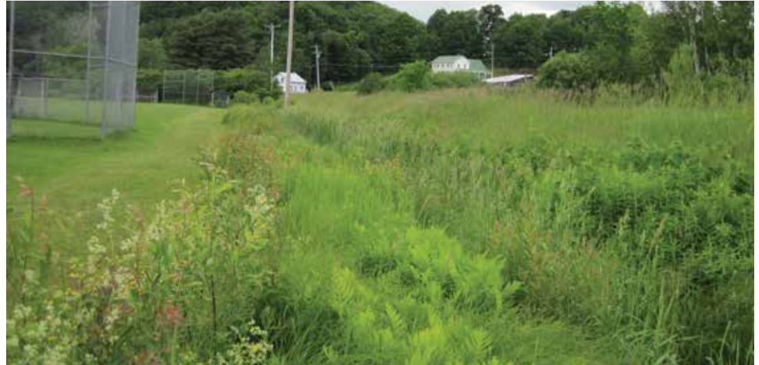
Vegetated swales allow water to soak into the ground as it moves instead of being stuck in a pipe.
