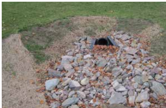
Diffuser stones slow down and spread out water as it leaves a culvert or roof downspout. Stones need to be greater than 3" in diameter and often greater than 12" at the end of a culvert where water is moving quickly.
