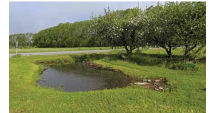
Raingarden after it rains
