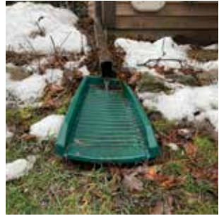
Downspout directed to lawn with end piece to spread water
