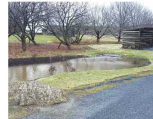
Driveway regraded to direct water to raingarden
