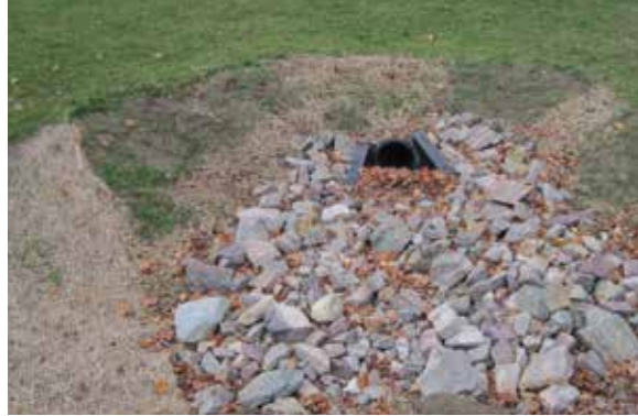
Diffuser stones slow down and spread out water as it leaves a culvert or roof downspout. Stones need to be greater than 3" in diameter and often greater than 12" at the end of a culvert where water is moving quickly.
