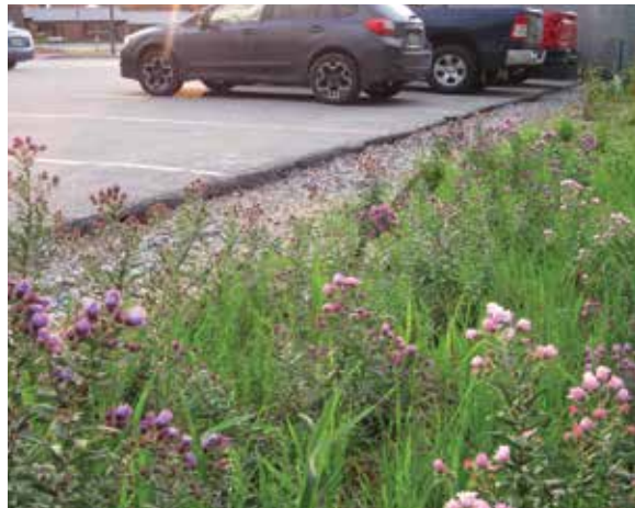
Stone level spreaders allow water that otherwise runs directly off the parking lot into the swale to drop into the stones and spread out.
