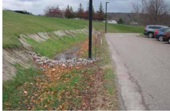
Check dams slow down and hold back water as it travels down a swale.
