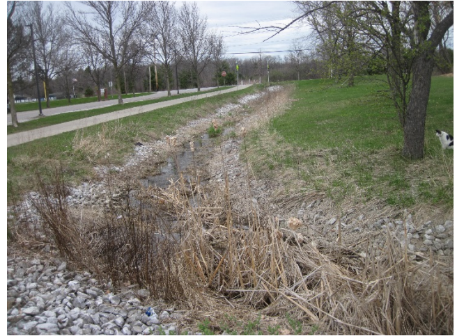
Figure 7: The swale continues parallel to the school access drive where it enters a pipe along Harbor Road.
