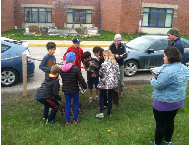
Figure 1: Students and engineers together inspect an existing catchbasin in entrance Island at front of school that currently drains through pipes directly to McCabes Brook.
