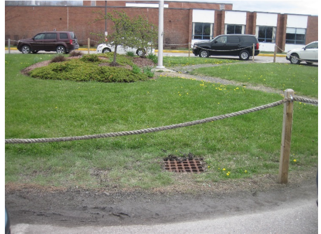
Figure 3: A close-up view of catch basin in the entrance island at front of school that could remain as the overflow from a bio-retention area.
